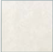
Polished Plaster to Ceiling
